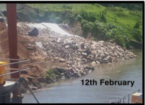
It appears this bank "stabilisation" is also resulting in a narrowing of the river at Thompson Square. In light of the sensitivity of hydrological conditions and the potential impacts on flood behaviour this is a matter of considerable concern.
